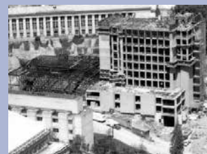
Ashe Auditorium and Chemistry Building construction at corner of Parkman Avenue and University Drive. Alumni Hall (now Eberly), in rear.
