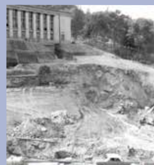
Excavation for Chemistry Building
